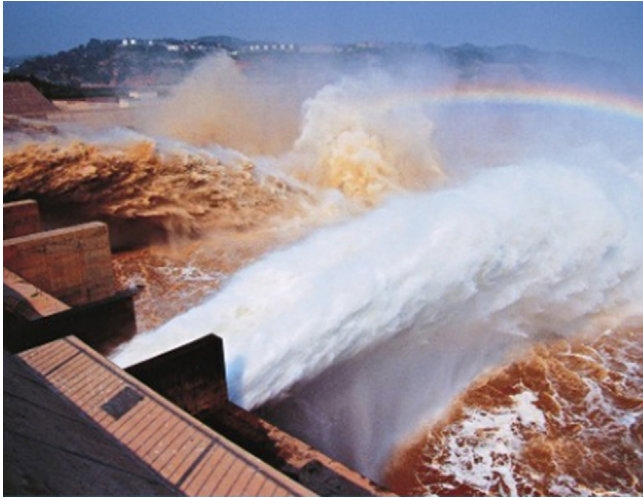
Fig. 7. Man-made flood generation in the Yellow River at Xiaolangdi, China. The highly sediment-laden flow scours the river channel over a long distance downstream.
