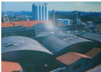
Figure 5.2: Aspect of the site, before the intervention
