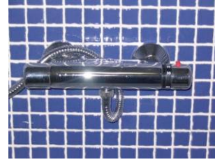
Figure 5.5: Thermostatic valves for the water temperature control
