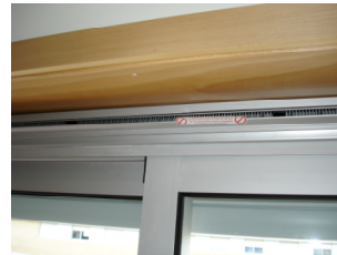
Figure 5.11: Self natural ventilated window frames
