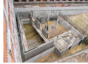
Figure 5.7: Underground water tank
