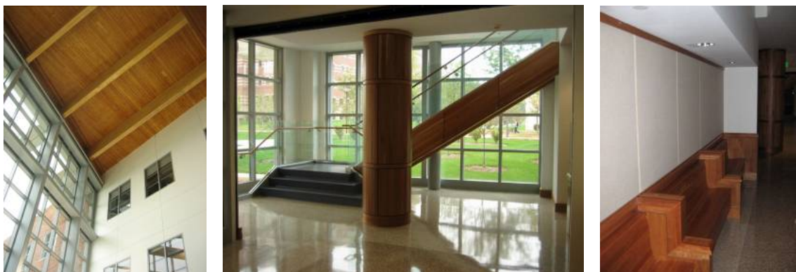
Figure 4-7: Locally-harvested wood on the Forest Resources Building
