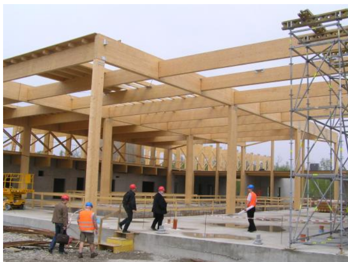
Fig. 3 UCEEB centre under construction
