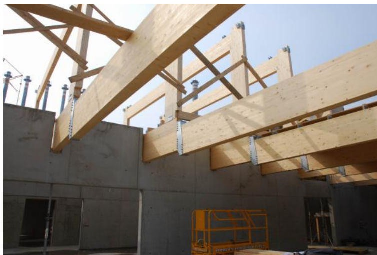
Fig. 4 UCEEB centre under construction
