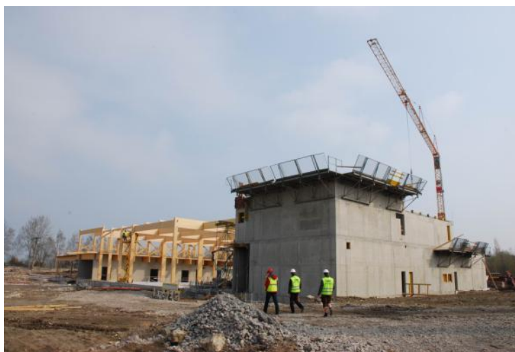
Fig. 2 UCEEB centre under construction
