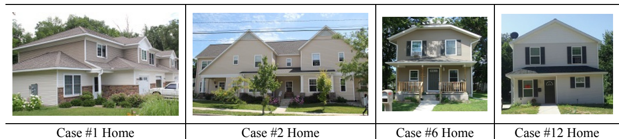
Figure 2. Photos of four case study Habitat homes
