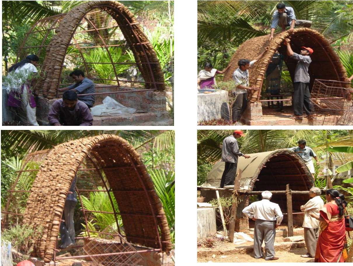
Fig3-6: Construction of Coconut shell sandwich panel structure- 4 stages
