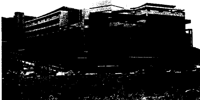
29.3 The view from the south-west, with the glazing and shading arrangement evident, and the canopy roofs just visible on the top of each block. The main entrance is to the left on the southern façade under the extended portico. The vertical strip of glazing punctuating the southern façade indicates the location of the atrium and the thermal flue can be seen above
