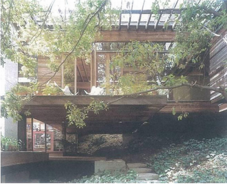
Fig. 10.32 Minimising the footprint of buildings on natural landscape (Yu et al. 2008b)
