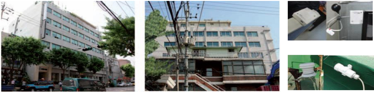
Fig. 2. Investigated building and monitoring equipment Equations
