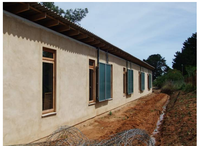
Figure 8. North facing wall with solar panels.
