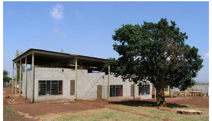
Figure 1. View of Khanyisani preschool in Orangefarm
