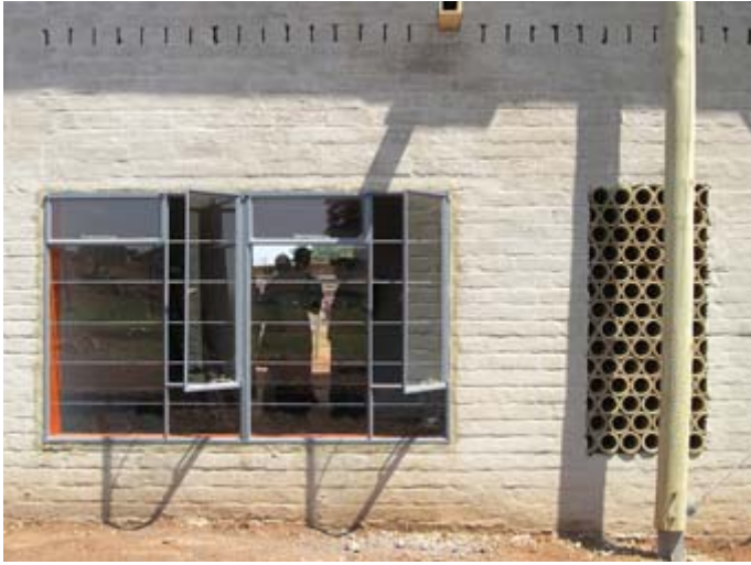
Figure 6. Playroom window in the North wall, screen made of wine-coolers on the right.
