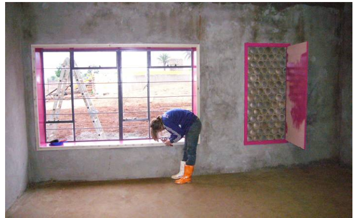
Figure 14. Inside view of window and shutter with screen at Khanyisani preschool
