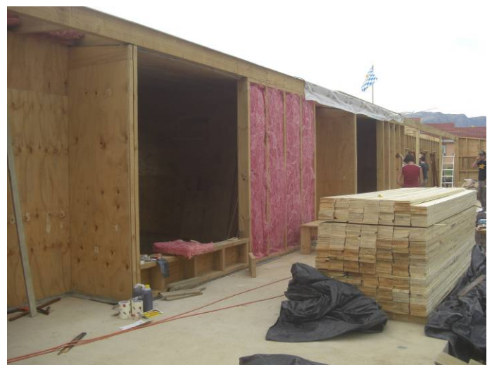
Figure 11. Insulation of the timber framed walls.
