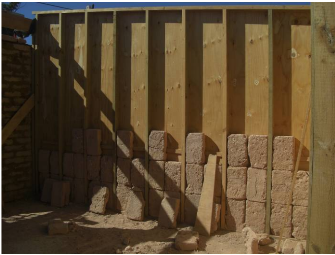
Figure 12. Clay brick filling of the partitioning interior walls.
