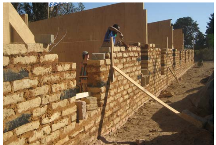
Figure 13. Brick laying, north wall.
