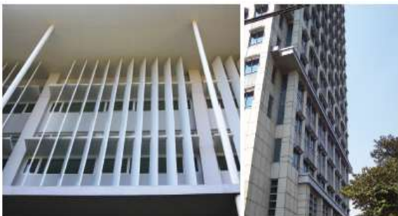
Figure 8. Example of the Vertical Fins Application (top left) (Boyles et al., 2009), The horizontal Shading (top right) Wangsadinata & Suprayitno, 2008)
